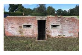
The Pill Box is an FW3/24 designed to be Bullet and Shell proof. The walls are about a metre thick, brick shuttered with reinforced concrete core.
